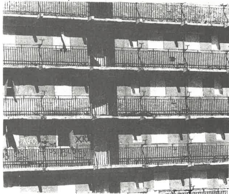
LIVERPOOL - A post-war block of flats, ready for coming down.
