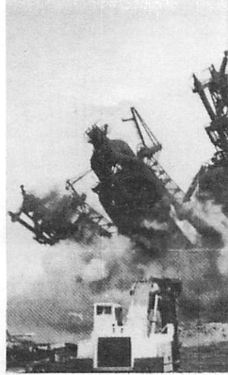
Demolition of a U.S. steel plant in Youngstown, Ohio.
