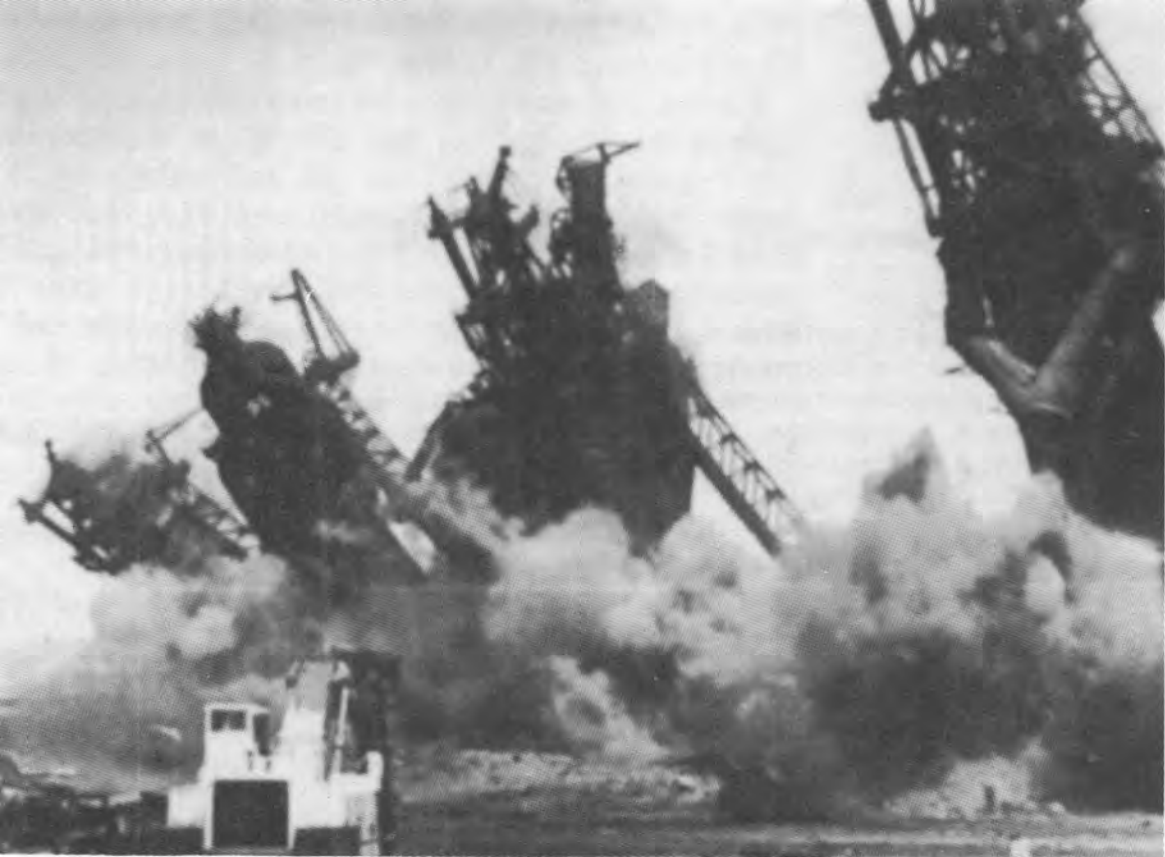
U.S. Steel blast furnaces being blown up after plant shutdown in Youngstown, Ohio.
