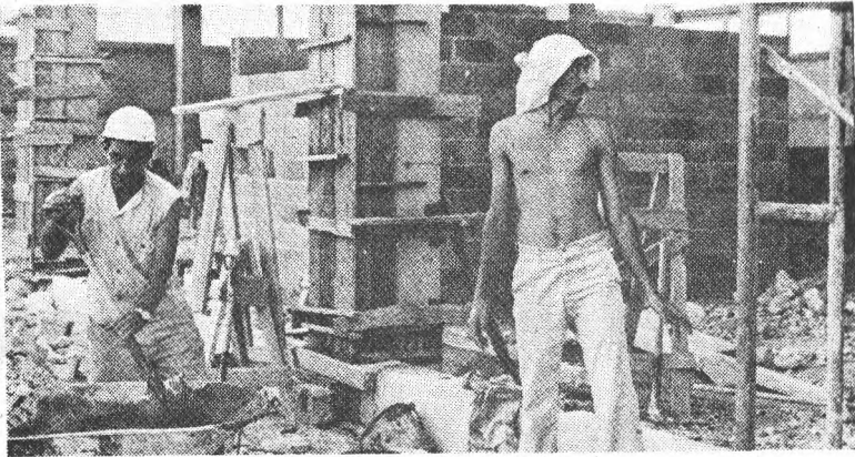
Construction workers in La Habana
