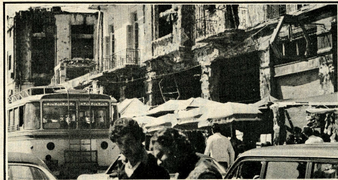
The long fighting in Lebanon has left its scars on the face of the cities and countryside. The capital city of Beirut has been damaged in the continuing civil war. Commercial buildings and private homes alike were demolished when the Zionists shelled the coastal city of Tyre during the most recent invasion.
