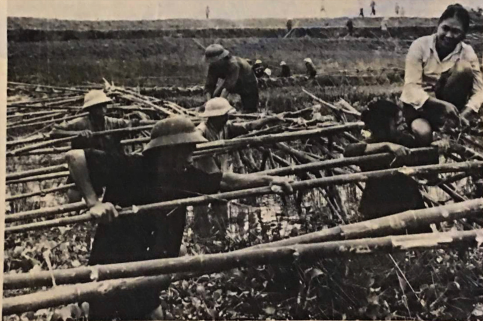
Workers of an engineering factory in Nam Ha in the Red River Delta building dams against floods.
