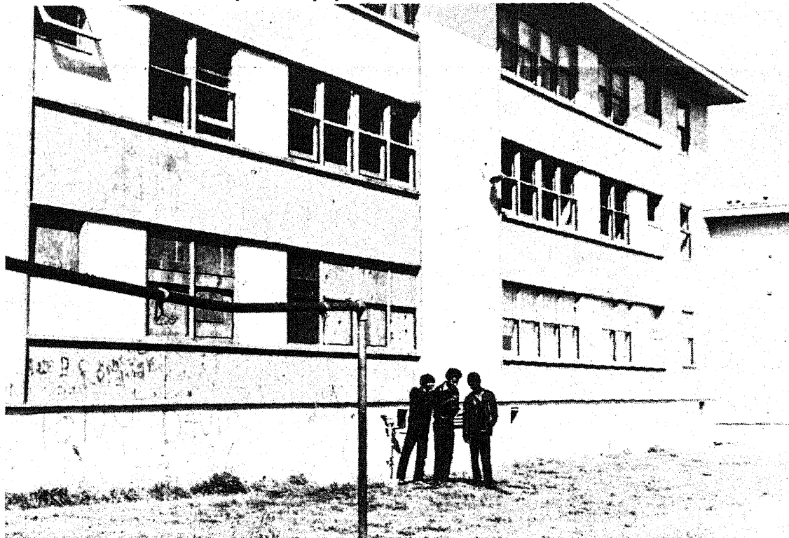
Rents are going up for Hunter's Point residents while Housing Authority allows deteriorating conditions.
