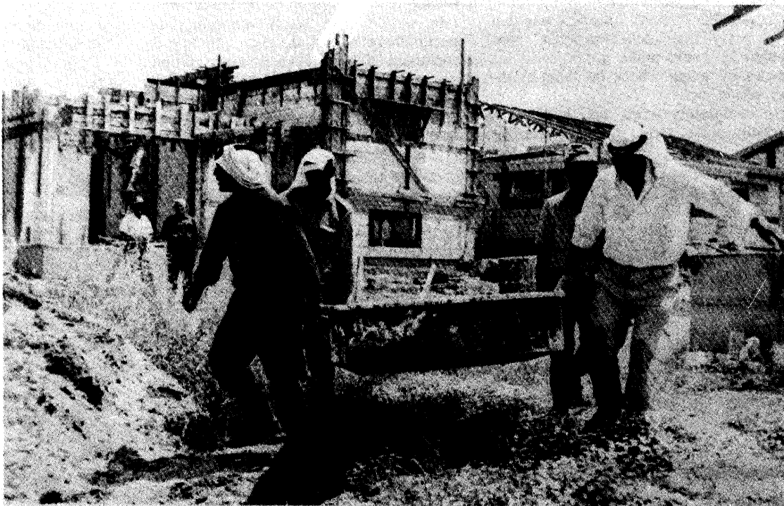
Arabs working on construction in occupied territory.
