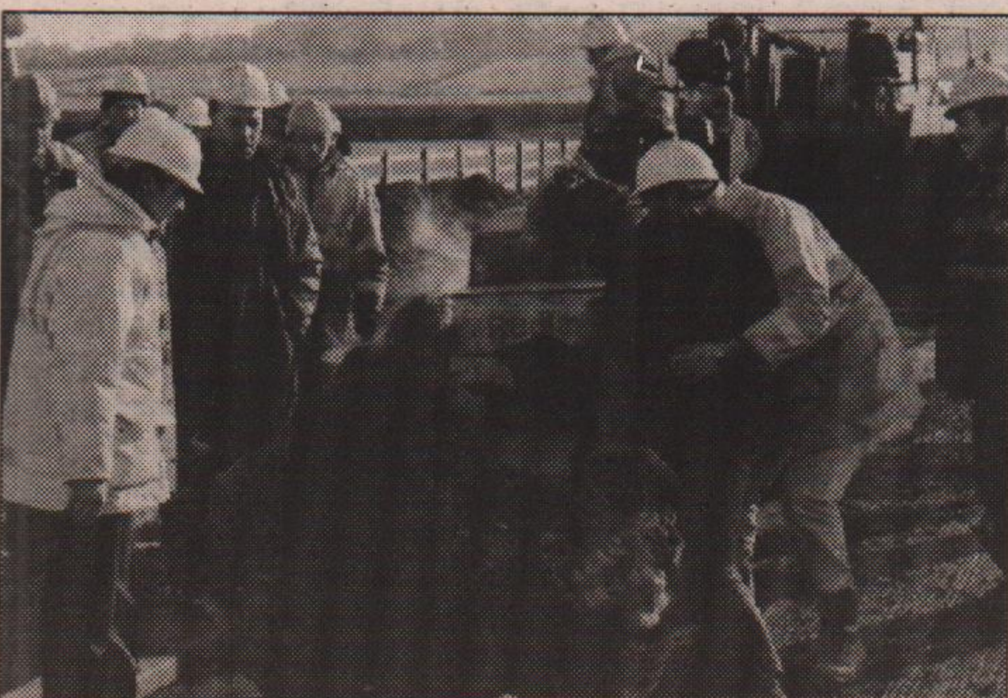
Leadenham bypass - protesters halting work on the site
