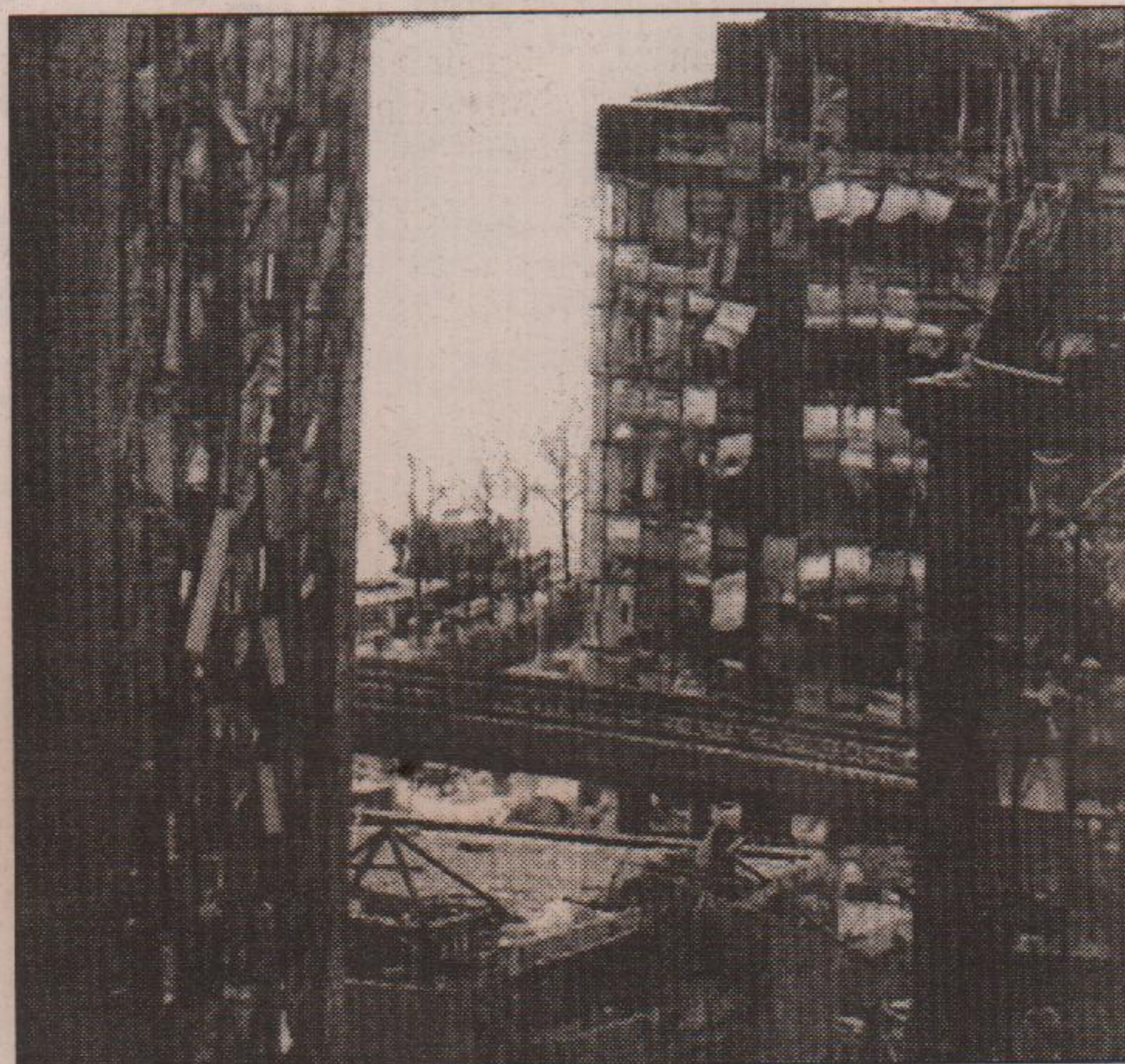
Massive damage at Canary Wharf
