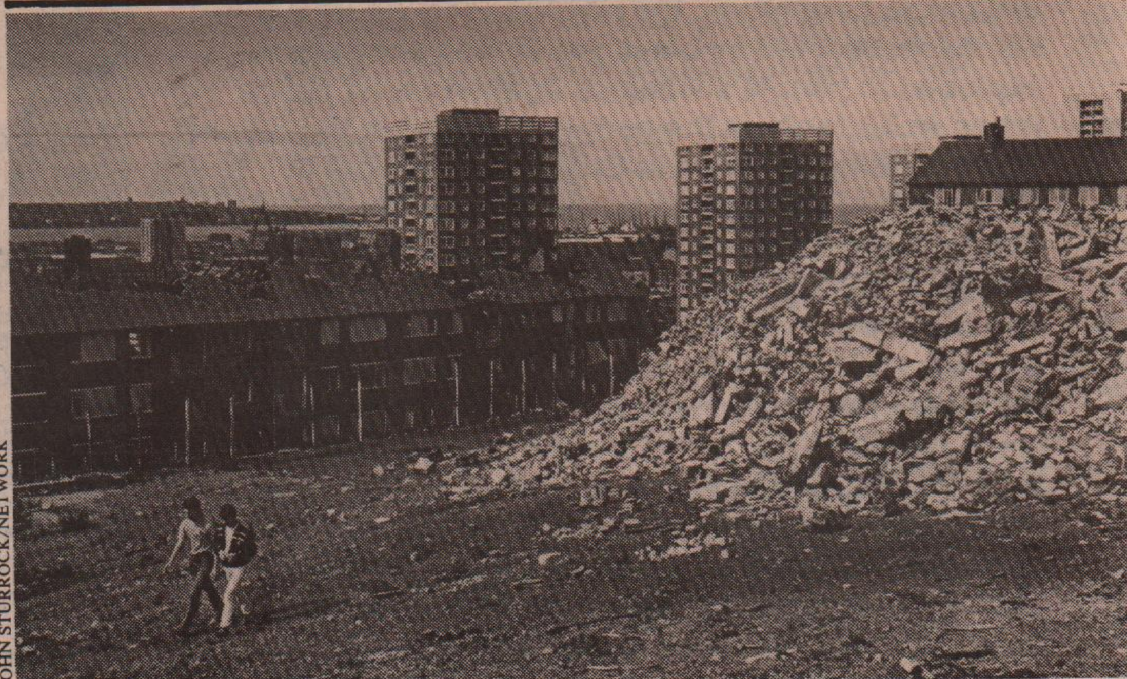
Demolition taking place in Urban Regeneration Scheme
