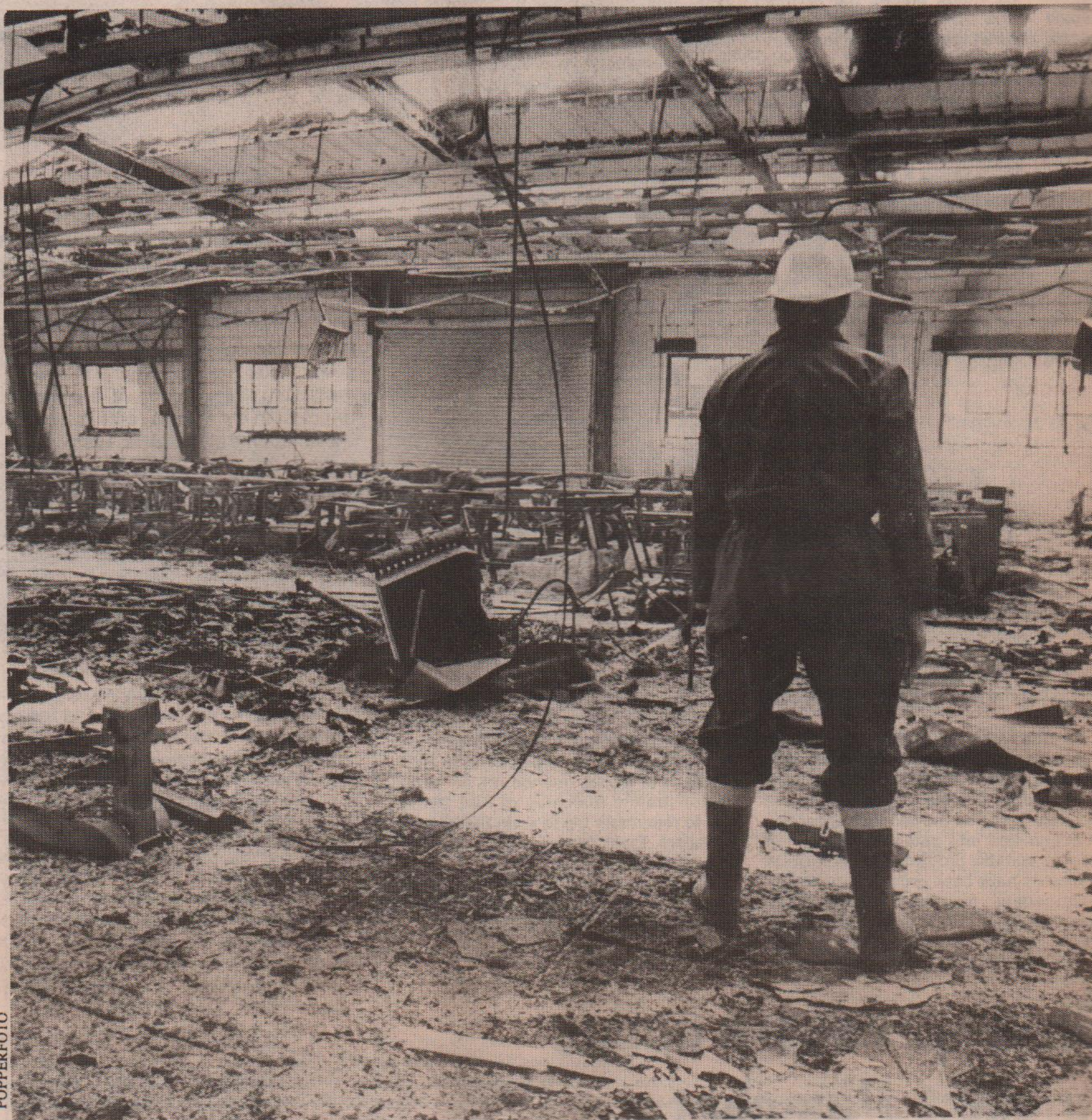
Northeye prison at Bexhill, burnt to the ground
