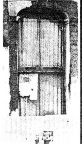
Boarded up house in Britain: all too typical
