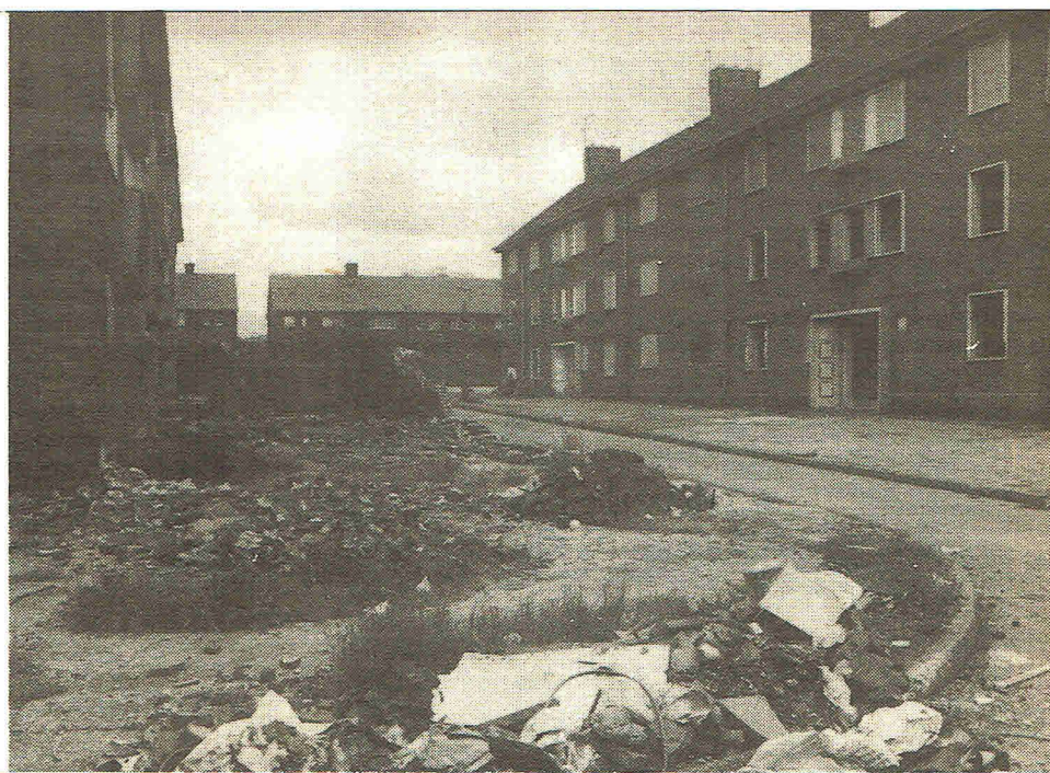
Maisonettes in the Vauxhall area of Liverpool, due to be demolished if the Labour council are victorious. Some are still occupied
