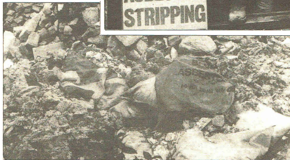
Above: Acre Mill near Hebden Bridge, Yorkshire, which suffered widespread asbestos pollution. Right: Worker at Lancaster Moor Hospital without protection against asbestos dust. Below: Asbestos dumped on a rubbish tip in Lambeth.
