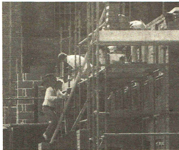
Some of Liverpool's new housebuilding.
