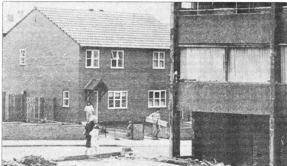
One of the many new council estates goes up in the shadow of "The Piggeries" a notorious high rise slum due for demolition shortly.
