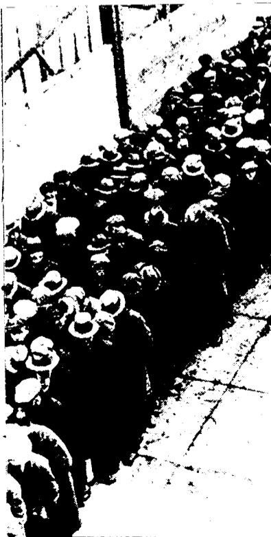
A new devastating slump
