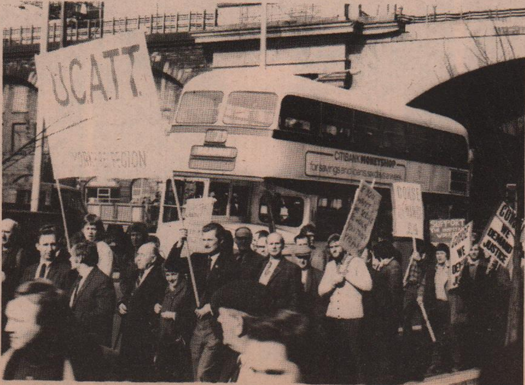
'We can't win on our own'... Sheffield building workers on a hospitals march
