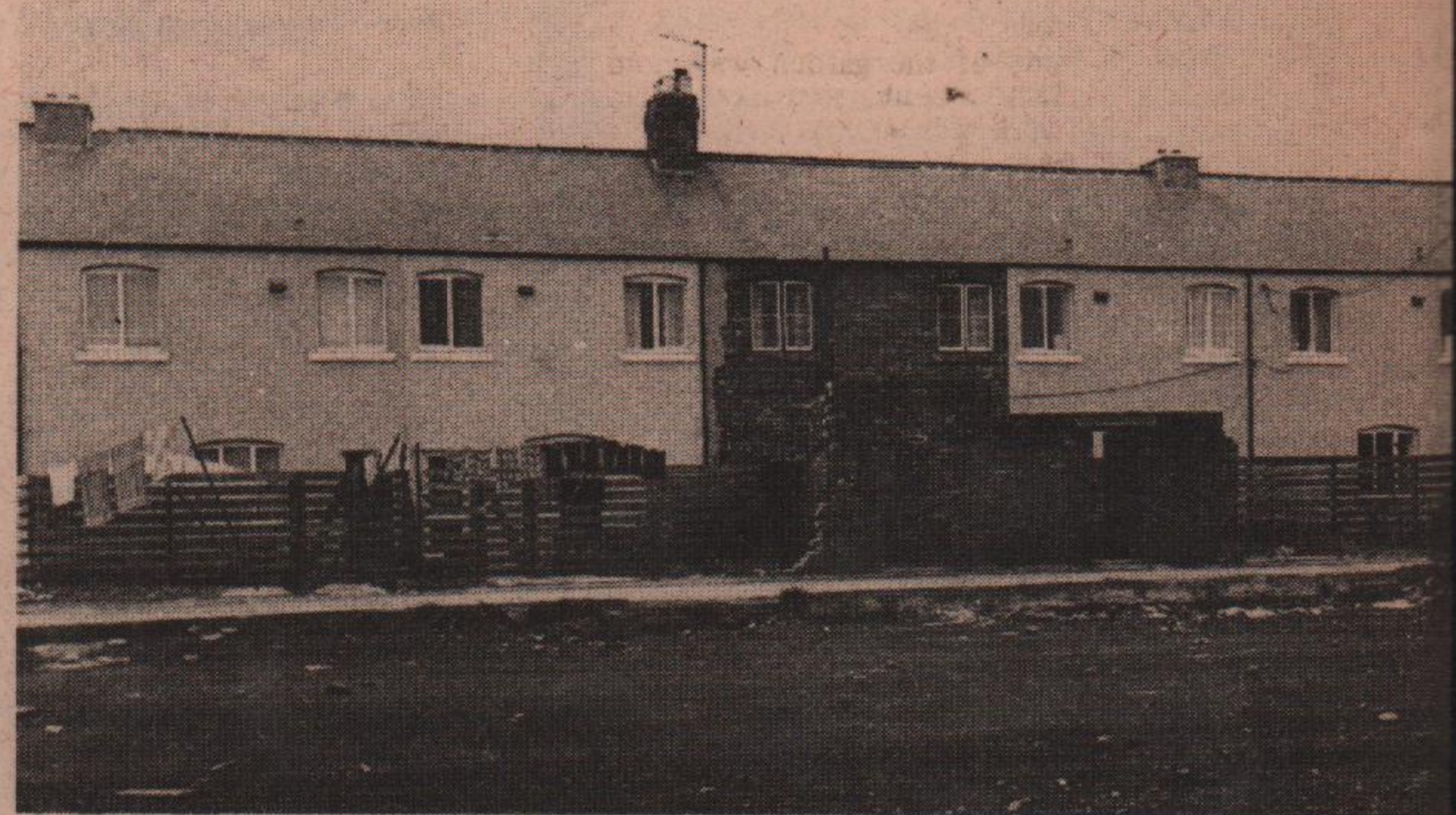
Bristol Street, New Hartley, 'revitalised'.
