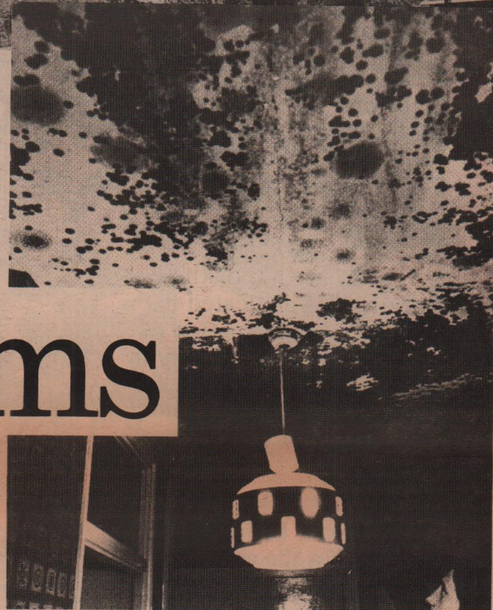
The old slums come slowly down in Coventry—but the new high flats are a grim alternative. Above is the ceiling of a flat on the Wood End Estate mottled with damp. A complaint was made a year ago but no action has been taken.
