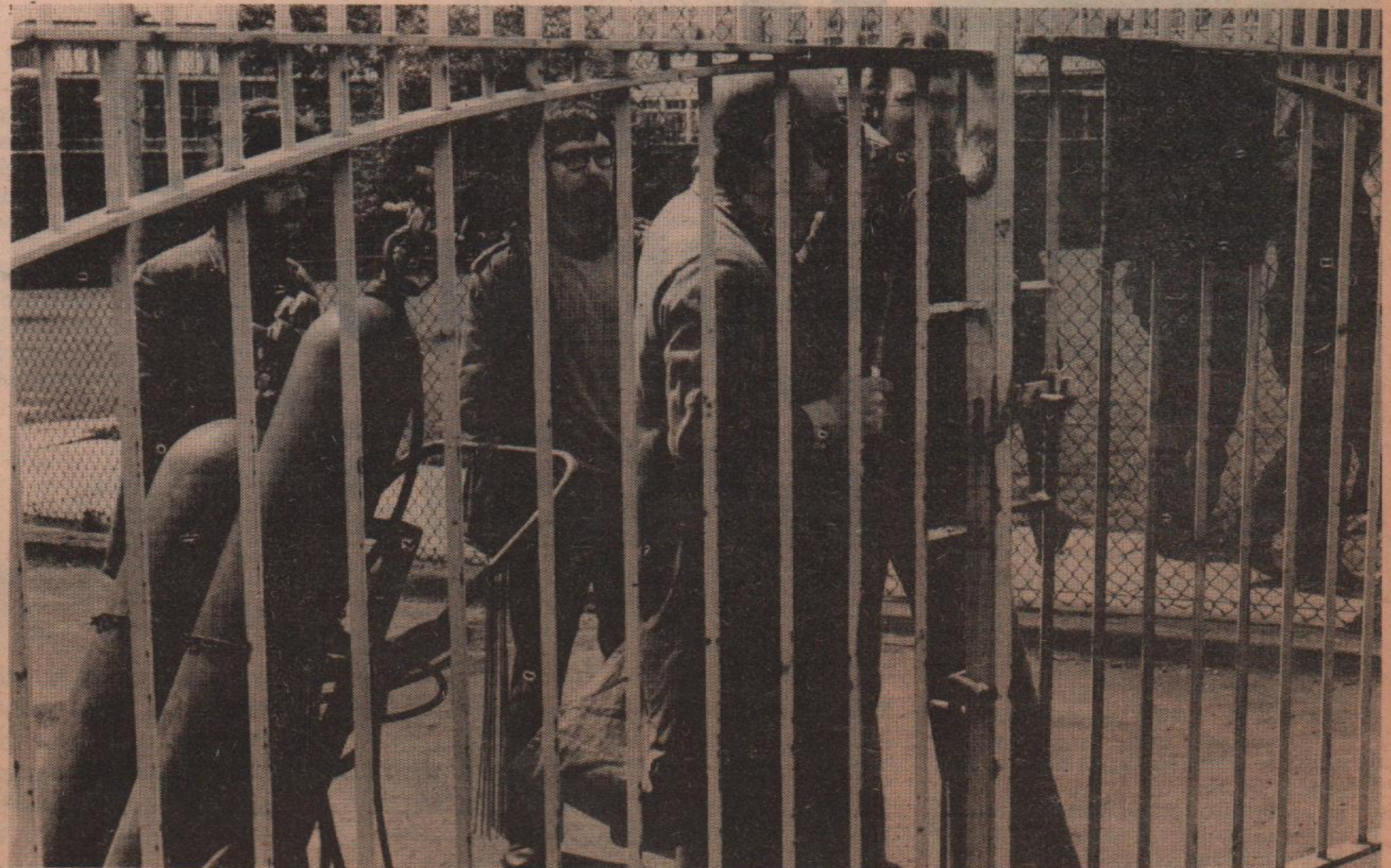
Welding the gates for the second occupation in two years. Picture: Ron McCormick. More pictures — page 9.
