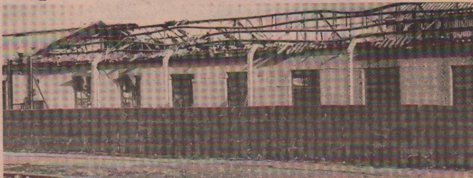
The San-Mex factory; it was production as usual the very next day
