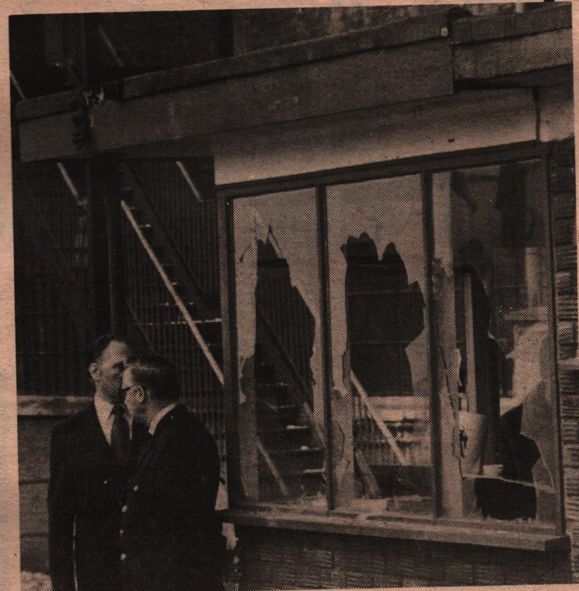
Broken windows and (Top) overturned Post Office vans: the scene after last week's explosion
