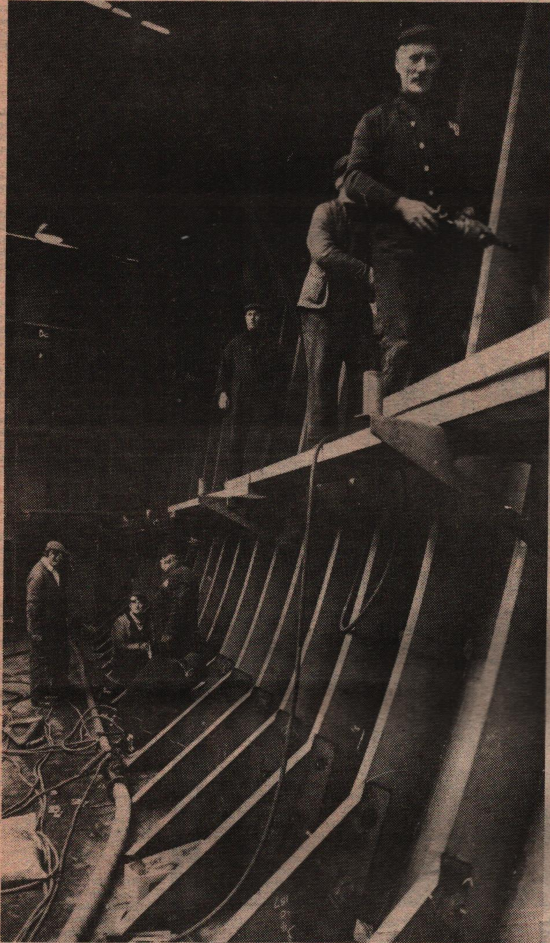
Welding and riveting inside a ship's hull: 'When the welding starts we all start choking.'
