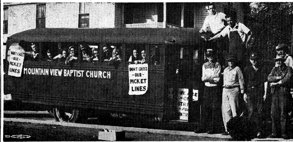
In Tuxedo, North Carolina, a company town, workers of the Green River Mills can't get a meeting hall. So the church bus, which they own, serves as union headquarters. The strike, led by the CIO Textile Union, has been on since April 6. Wages in mill averaged 87c. an hour. With little economic reserves, the strikers are finding the going rough. Contributions for these strikers are welcomed by the CIO-TWUA.
