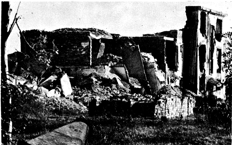
A house destroyed by U. S. bombing raid in Vinh region of North Vietnam.
