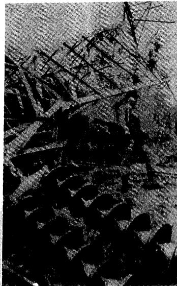
Government soldier stands guard over remains of electric power line tower toppled by FMLN.
