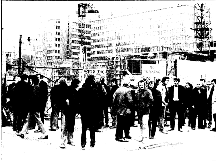
Building workers picket McAlpine's
