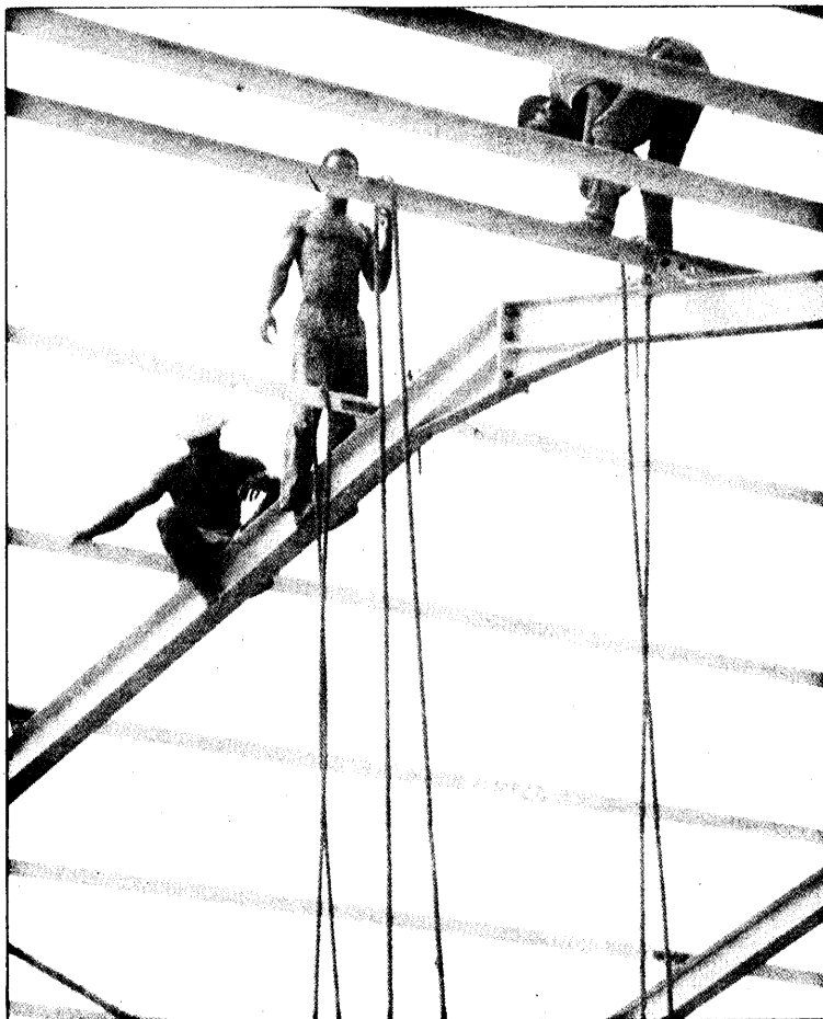
Factory building for Dorman Long who are reaping the benefits of investing in apartheid. Above: living conditions of black workers.
