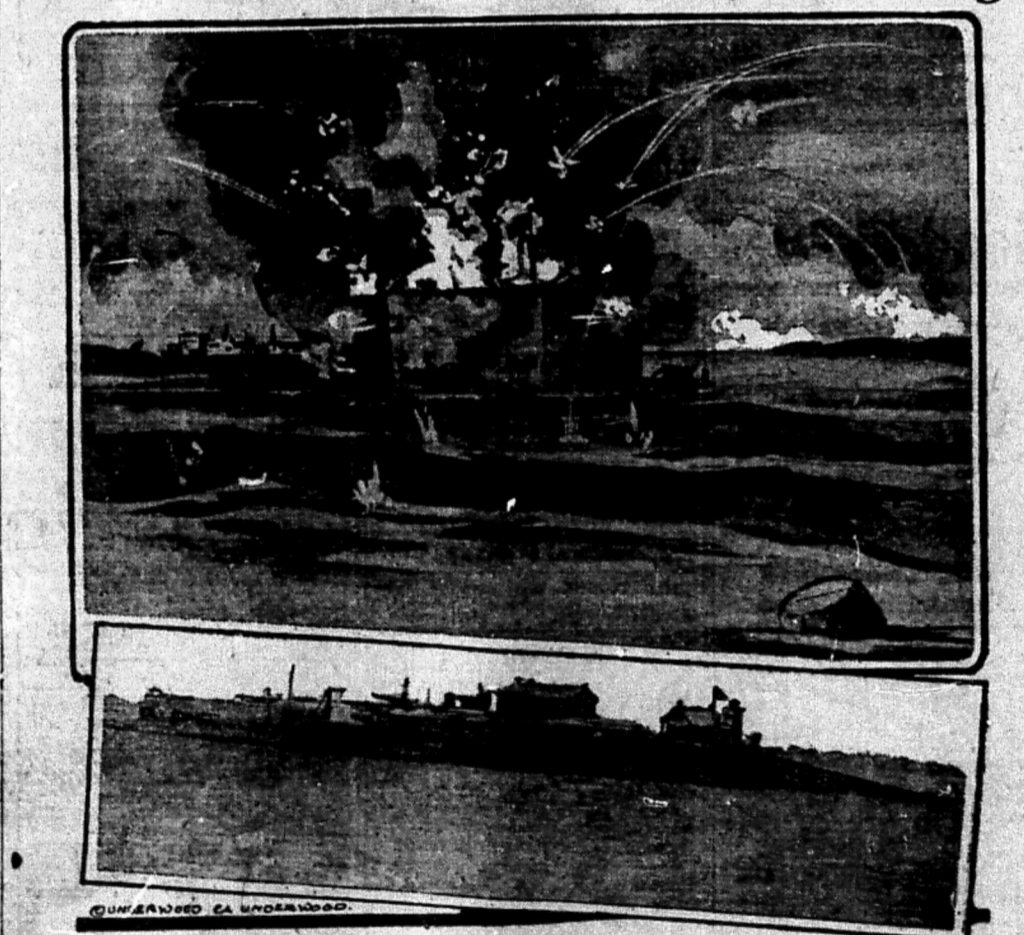
AT TOP, A WARTIME PICTURE OF THE BOMBARDMENT OF FT. SUMTER ON APRIL 12, 1861. BELOW FT. SUMTER AS IT LOOKS TODAY.
