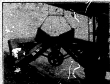
NEW GRAB BUCKET HOLDING SEVEN AND A HALF CUBIC YARDS AND SPREADING TWENTY FEET. NOTICE RAILROAD RUNNING UNDERNEATH.
