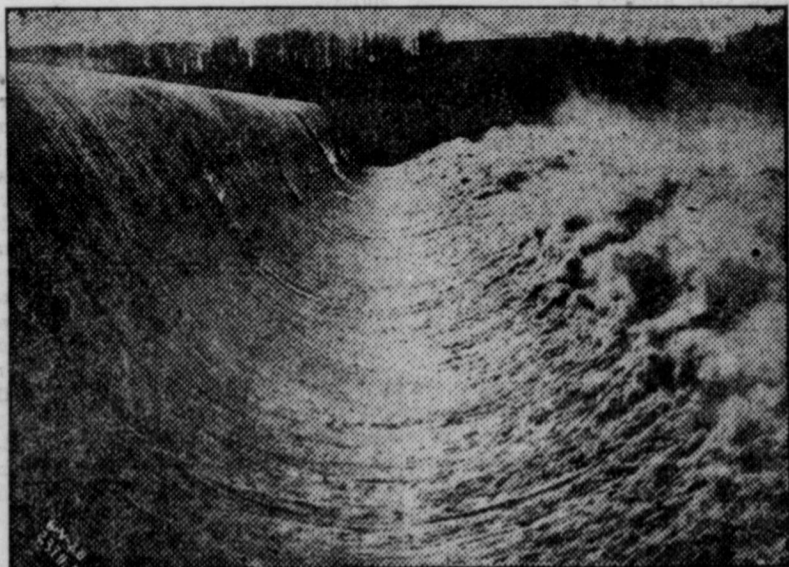
Volkhovstroy Dam, 30 ft. high, 290 ft. long.
