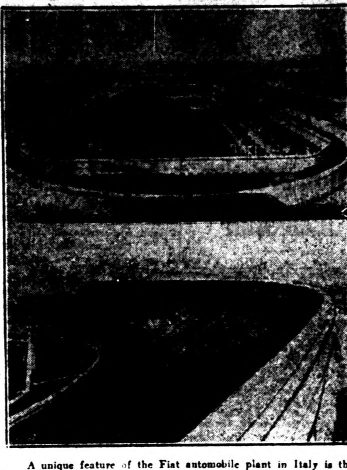
A unique feature of the Fiat automobile plant in Italy is the roof race course on which both racing and stock cars made within the structure are tested. The track is of concrete, with high banked turns, as can be seen from these photos.
