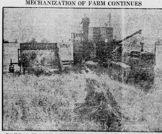
New Holt caterpillar grain harvester, picks up bundles, cuts strings, threshes, and cleans grain in one operation, thus eliminating all of threshing crew except binder driver and shockers. It is an expensive thing for the individual farmer and will be bought with a mortgage on the farm, or by the local bankers and grain dealers and rented to the farmers, unless co-operatives are formed to purchase such machines. THE DAILY WORKER, NEW YORK, TUESDAY, NOVEMBER 22, 1927
