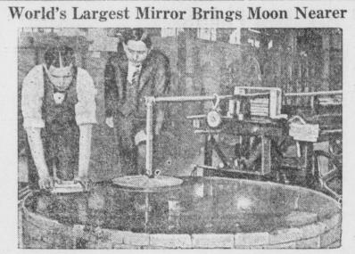
This 70-inch reflector, the largest mirror in the world, is now being completed at the Bureau of Standards. Photo shows A. H. Lindner, left, polishing the mirror under the supervision of A. N. Finn, right. When completed, the mirror will be placed in the telescope of the Ohio Wesleyan University.
