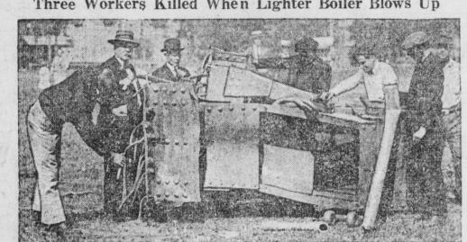
Two firemen and the engineer were killed and other workers were injured when the boiler of the steam lighter Chancellor, blew up recently. The picture shows the base of the boom which landed in a ball park 400 feet from the scene of the tragedy
