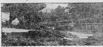
Washout of bridge where the waters of the Roundout Creek swept downward rush after heavy rains caused a flood.
