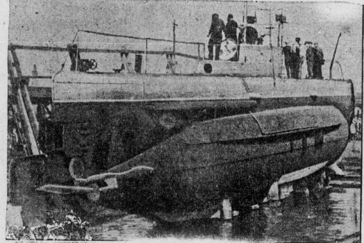
The latest instrument for slaughter in sea warfare is the above submarine defender, equipped with trap door to permit diver to leave and return while vessel is submerged.
