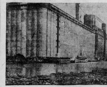
Terminal elevator at Port Arthur, Canada. The elevator into which flows much of the wheat harvested in western Canada, has a capacity of 6,900,000 bushels and represents an investment of \$5,-
