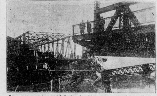
narrowly escaped death when the 1,000-ton eastern section of the Lincoln Highway Bridge over the Hackensack River suddenly collapsed. Improperty built supports—the work of the Jersey graft machine-were the cause of the collapse.
