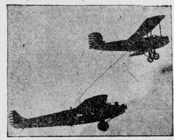
The U. S. Army's Fokker Plane, "Question Mark," which has now made a five day flight, breaking all previous records for any type of airship. Refuelling in midair is the secret. The plane is shown receiving gasoline thru a tube from a plane flying above it, while flying over San Diego, Calif. To the South lies Mexico, much nearer than five days away, and south of that, within range of the new flight power, all South America.
