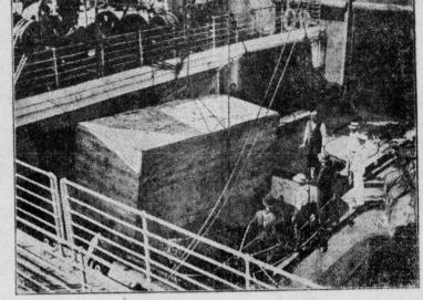
lowering a boxed auto, a heavy load, to a pier. The gangway man steadies it with a touch of his hand. Note open hatch, down which dockers often fall, causing serious injury or death. The second photo shows dockworkers raising a load to the level of the hatch coamings.
