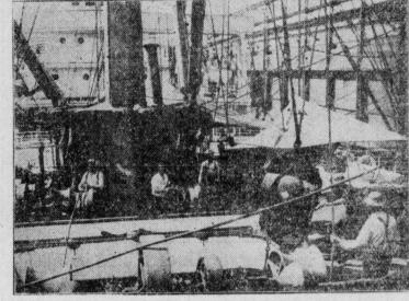
This load is one of 3,000 pounds. A load of barrels is being swung by the workers in the picture at right. These photos illustrate another danger to dockers, besides danger of being hit by loads and falling into open hatches-low hatch coamings.
