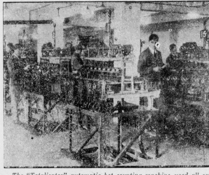
The "Totaliator" automatic bet counting machine used all over England and at Longchamps, France. Forty-two electric calculators at Longchamps show instantly the winning prices on boards outside.
