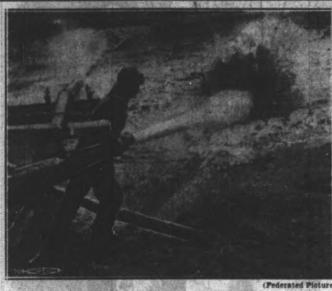
In the gold fields of the Soviet Far East the most improved methods of extracting gold from the soil are being used by the Soviet mining trust. The worker shown above is using a hydro-monitor to speed up -and efforts like his are making gold production in th
