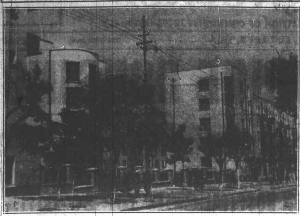
These homes are occupied by ship construction workers at Sevastopol, Crimea. Structures such as these are going up in all parts of the Soviet Union.
