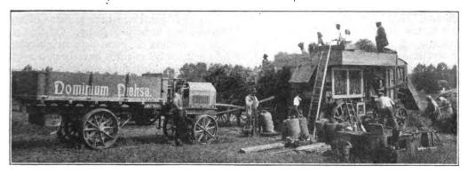
THE MOTOR OF A MOTOR WAGON DRIVING A THRESHING MACHINE.
