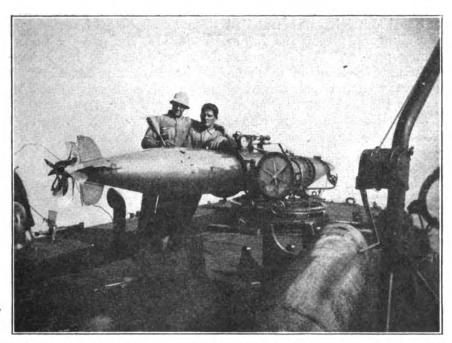
LOADING THE WHITEHEAD TORPEDO. THE TORPEDO COSTS ABOUT \$6,000. THEY ARE 20 FEET LONG, 18 INCHES IN DIAMETER AND WEIGH 2,200 POUNDS.
