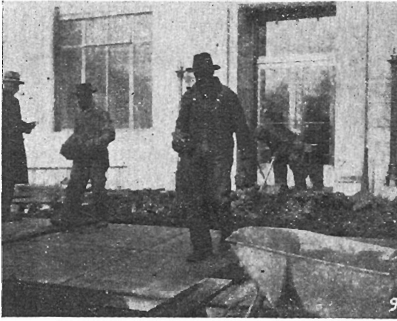
NEGRO WORKERS ON HOUSE WRECKING OPERATION
