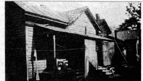
A typical Southern worker's shack, almost ready to topple over.
