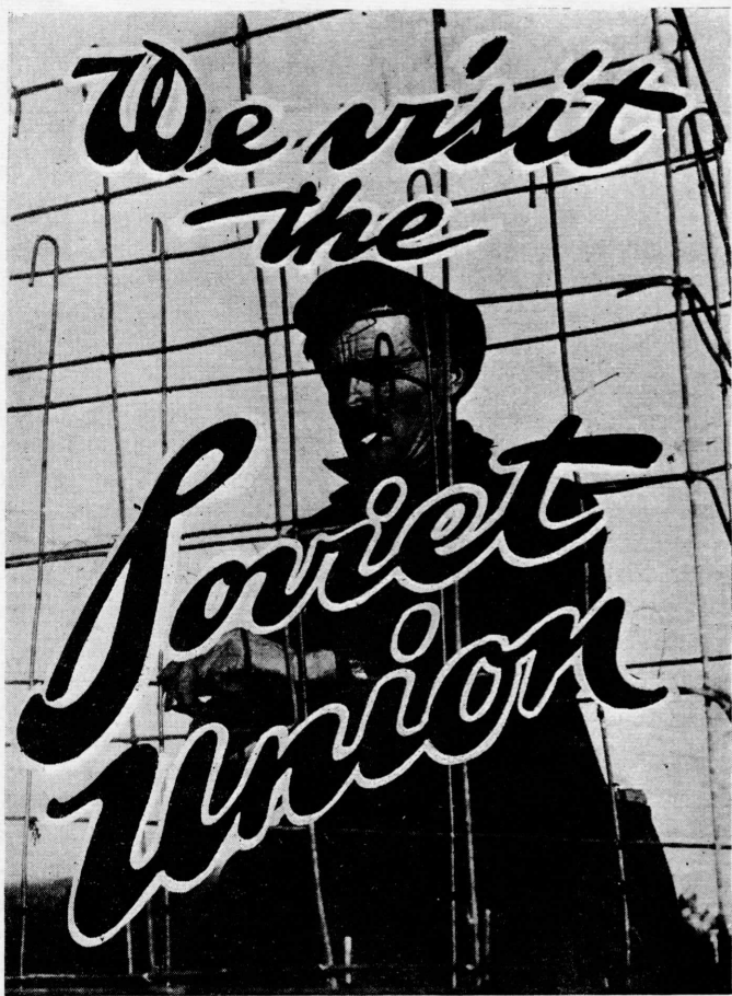
Constructing the giant cement combine in the Ural District
