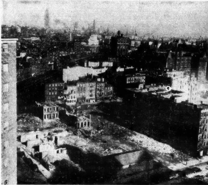
THIS IS THE LOWER EAST SIDE They learned how to work for better housing. . .
